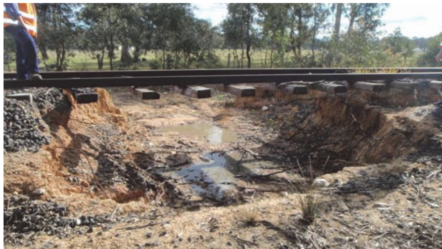
Figure 3B Pre-existing track issues on the Maryborough to Ararat line
