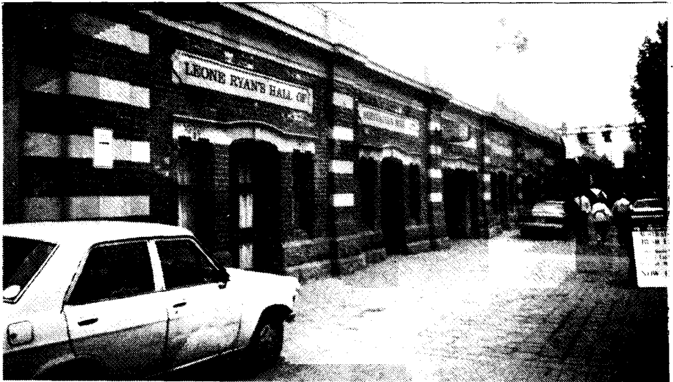
Banana Alley vaults, November 1988.
