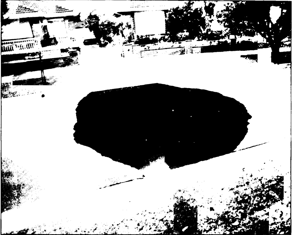
The Lawson Street, Moonee Ponds sewer collapse resulted in a hole 10 metres wide and 15 metres deep. (Photo: Courtesy of "The Age".)
