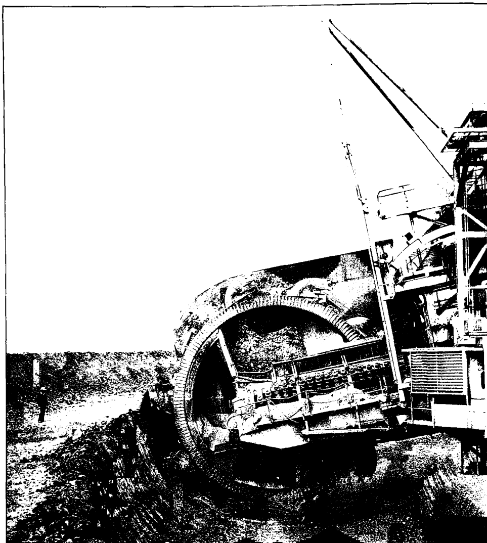
Overburden removal by bucketwheel excavation.
