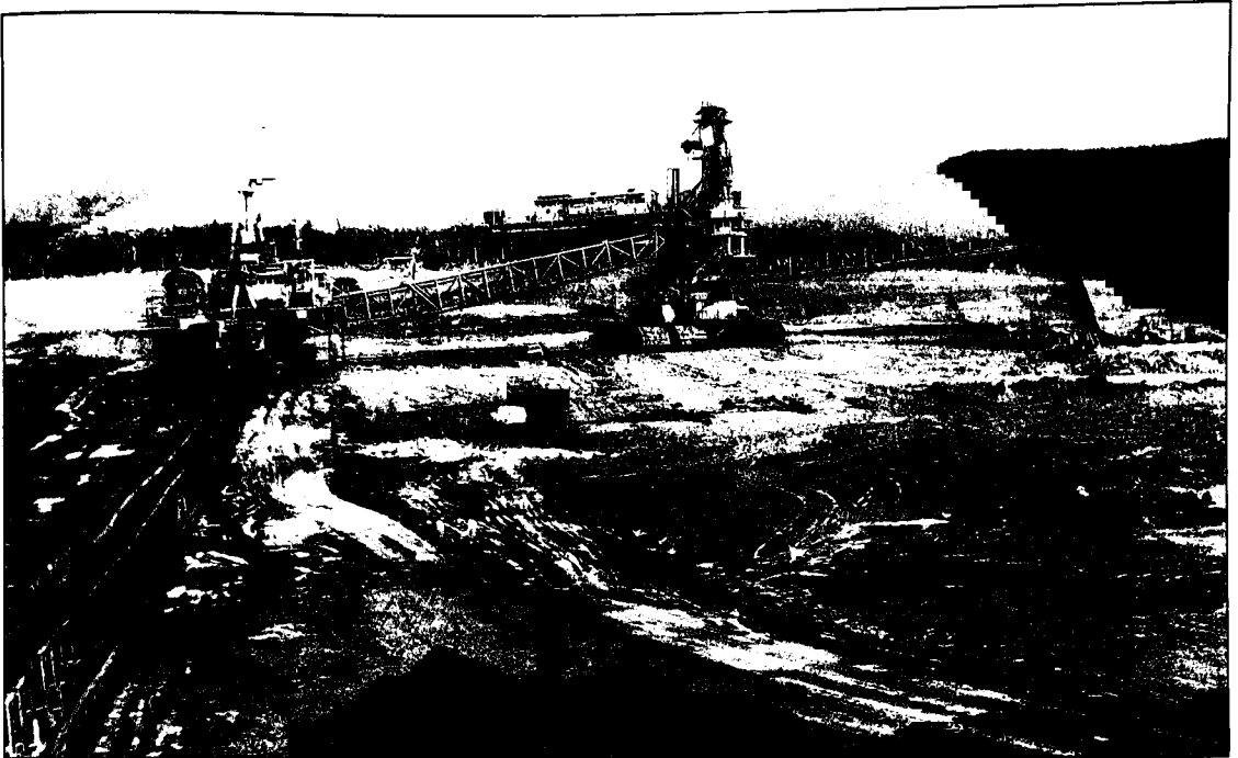
Travelling stacker depositing overburden.
