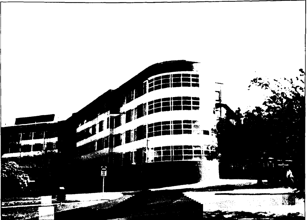
A large multi-storey geriatric centre.
