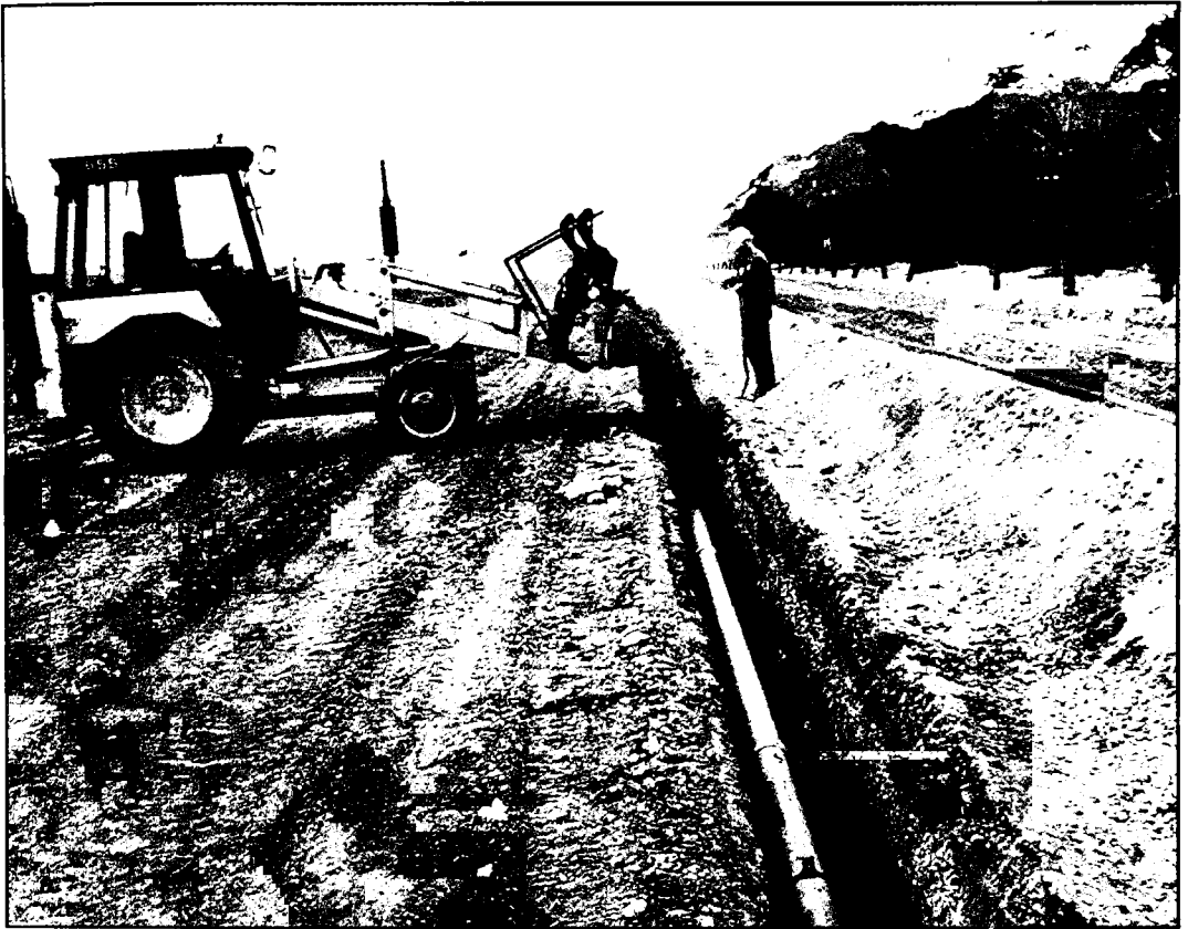
Laying of the Northern Mallee pipeline.
