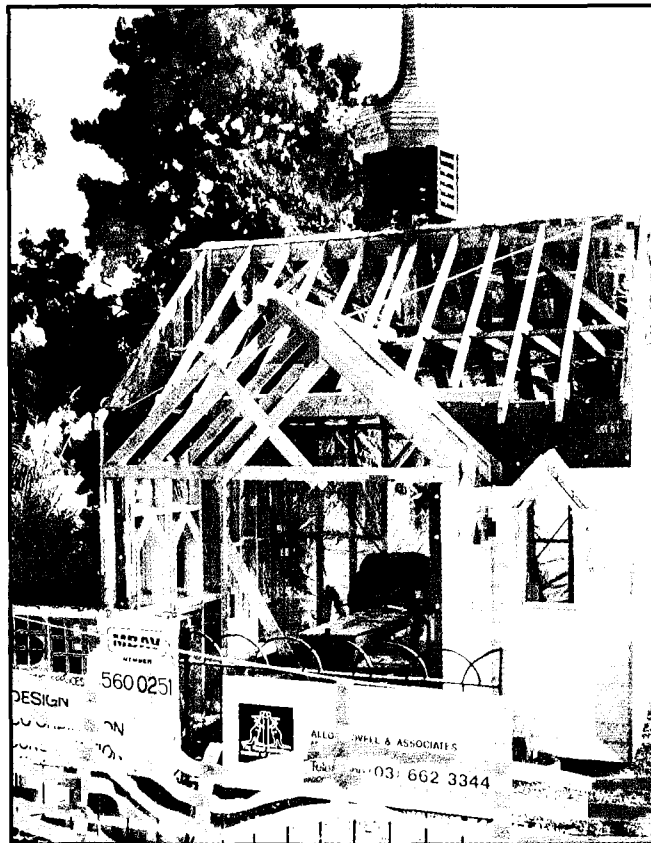
Reconstruction of William Tell Shelter following destruction by fire.
