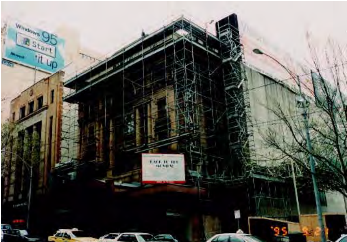
Regent Theatre during refurbishment.
