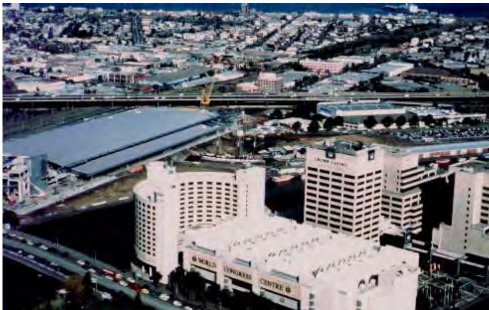
Melbourne Exhibition Centre and Melbourne Convention Centre located on opposite sides of the Yarra River.
