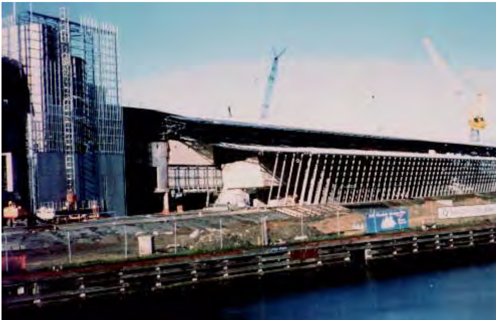
Melbourne Exhibition Centre under construction.
