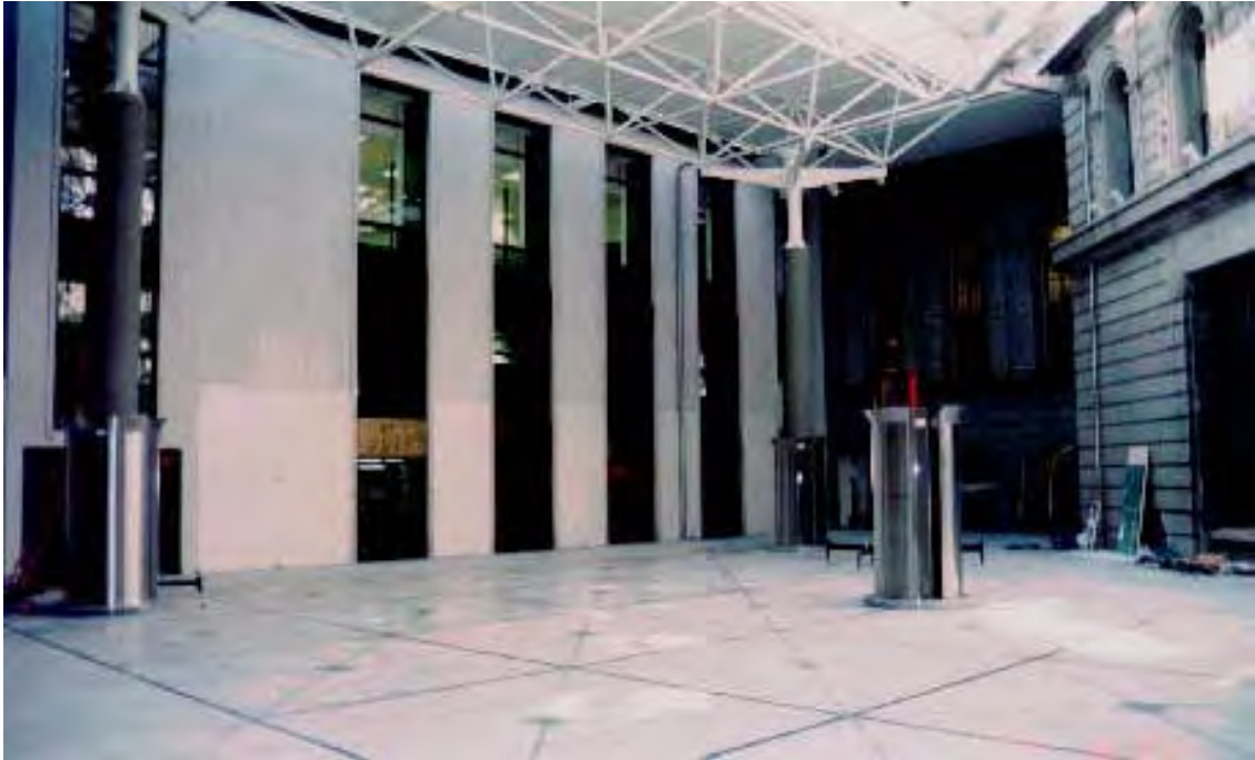
Completed North West Courtyard of State Library of Victoria.
