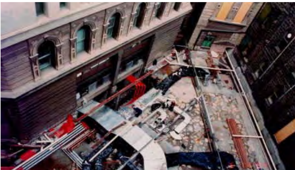
North West Courtyard of State Library of Victoria under construction.
