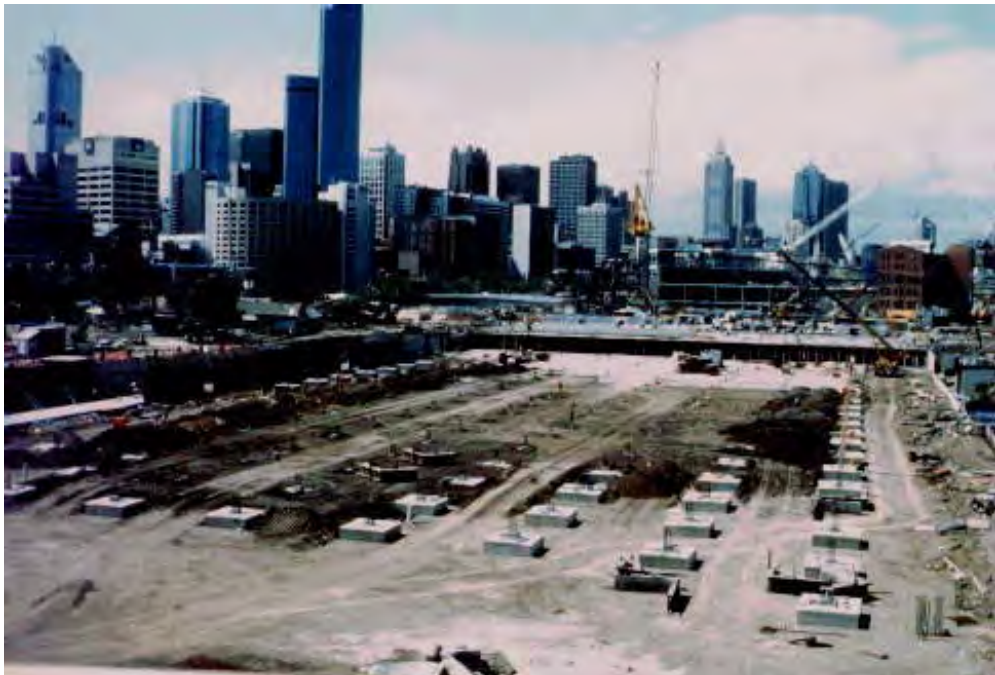
Construction site of the Melbourne Exhibition Centre.
