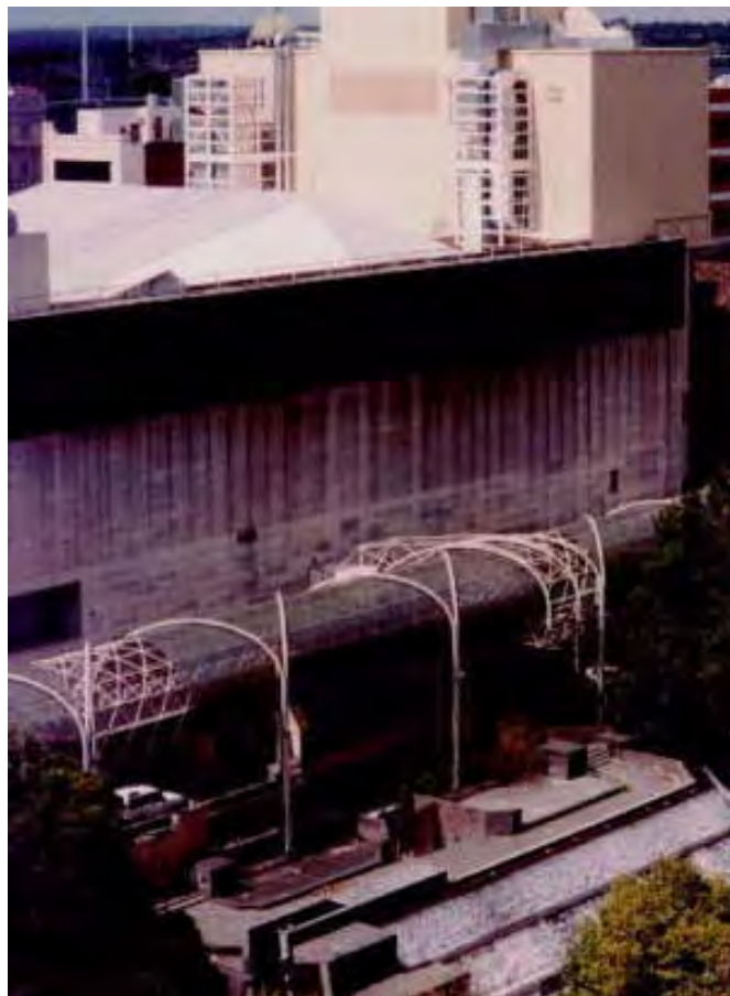
Completed Fly Tower Extension Works rising above the Regent Theatre.
