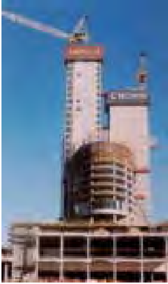
■ 1 Permanent Casino Under Construction
