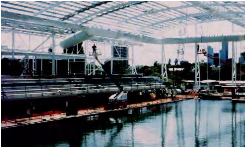
Pool area of Melbourne Sports and Aquatic Centre under construction.
