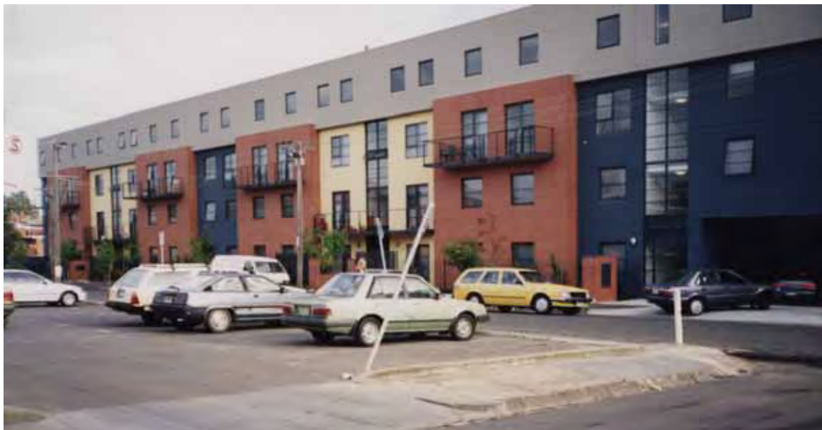
Car park and student residence complex, Hawthorn campus.
