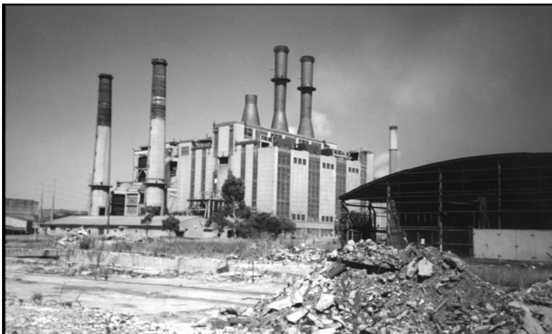
View of the Yallourn Power Station clearance work.
