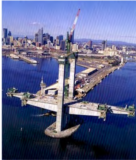
Construction works for new Yarra Bridge.
