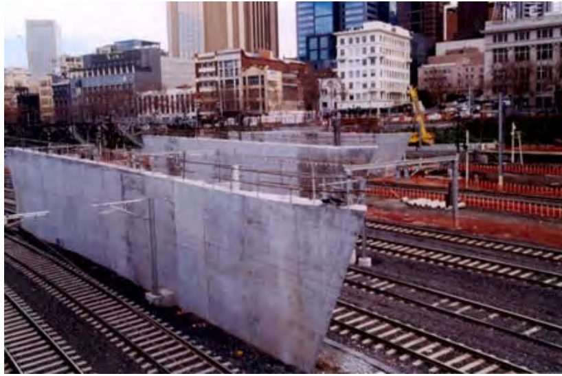
Exhibition Street extension bridge supports.
