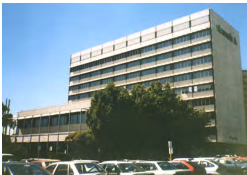
Former VicRoads property, Carlton.
