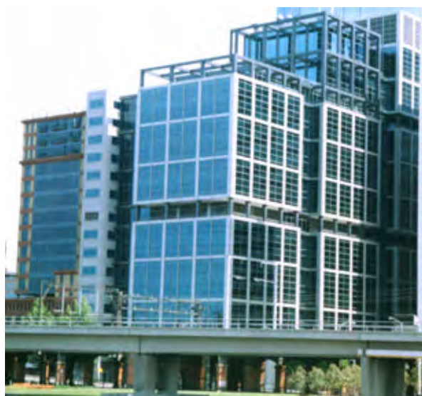
Former SECV building.
