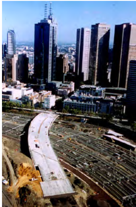
“City end” of the Exhibition Street Extension works.
