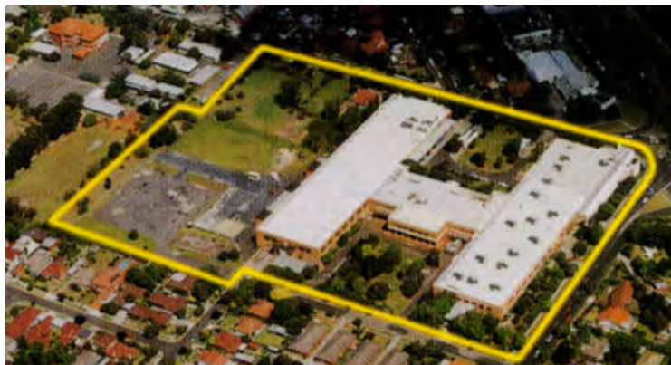
Aerial view of the Bentleigh site.
