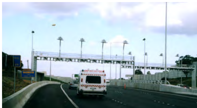
City Link tollway detection gantry.
