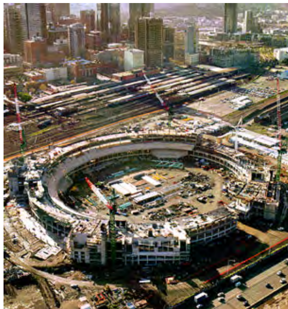
Docklands Stadium under construction.
