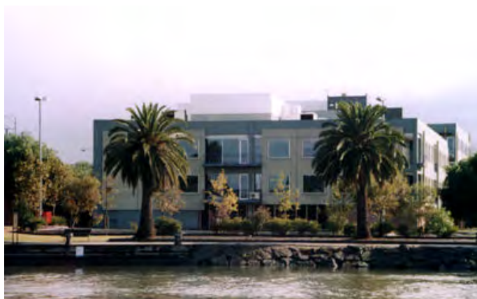
Office building constructed as part of the Quay West Project.
