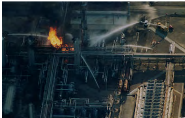
The September 1998 explosion and fire at the Longford processing plant. (Photo courtesy of The Age.)
