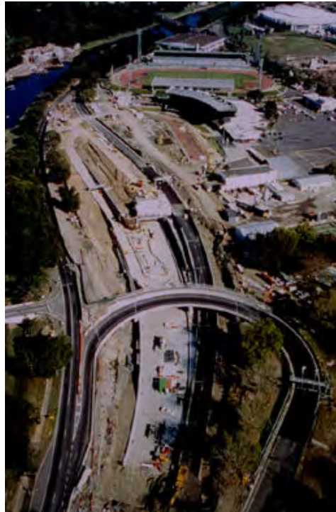
Exhibition Street Extension works, "Punt Road end".
