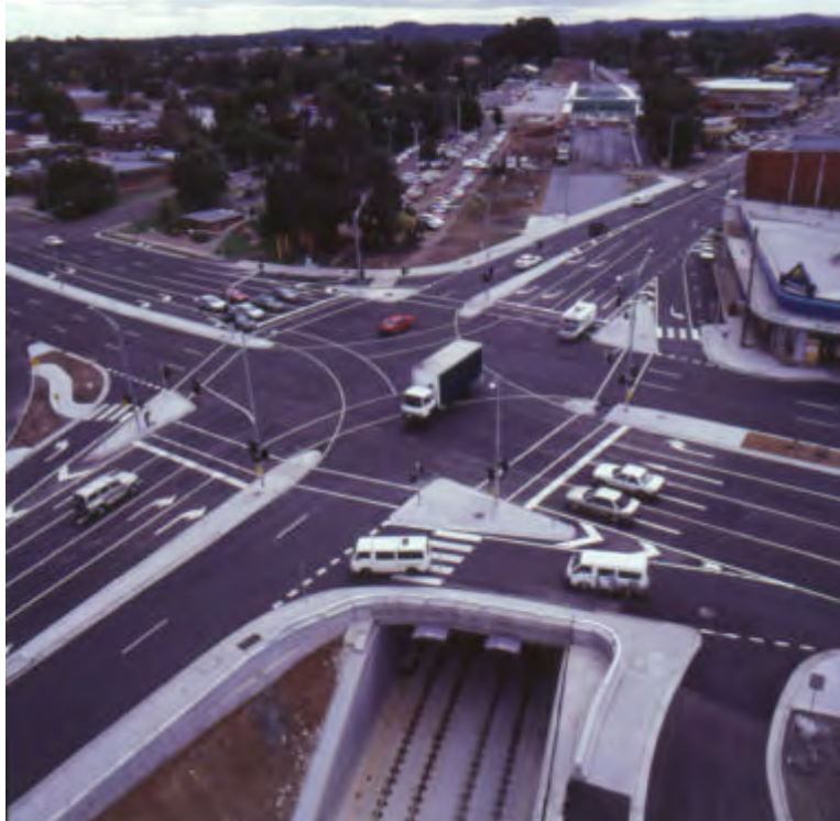
Completed rail and road traffic management project at Boronia.
