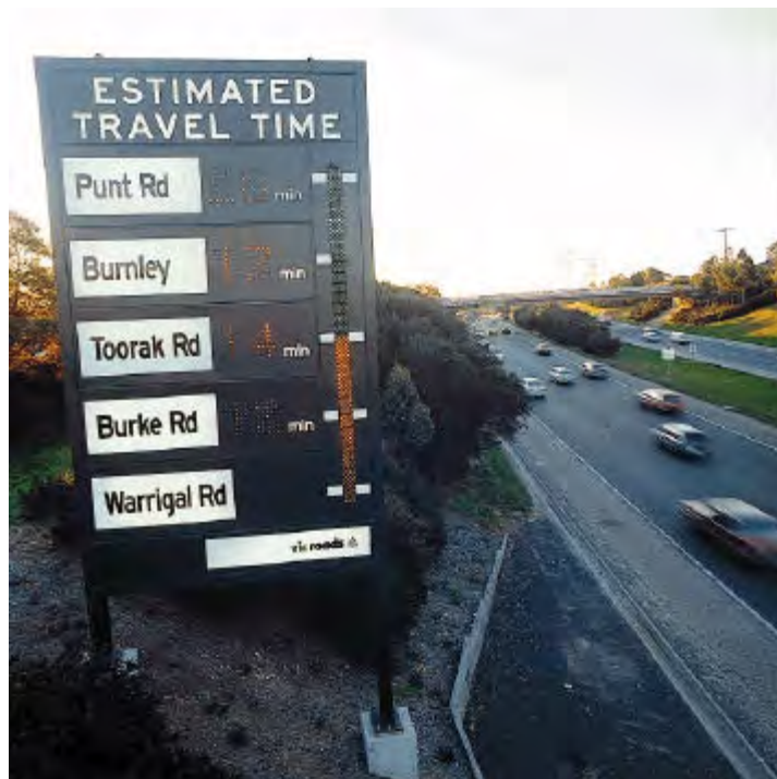
Travel time indicator on the South-Eastern Freeway.
