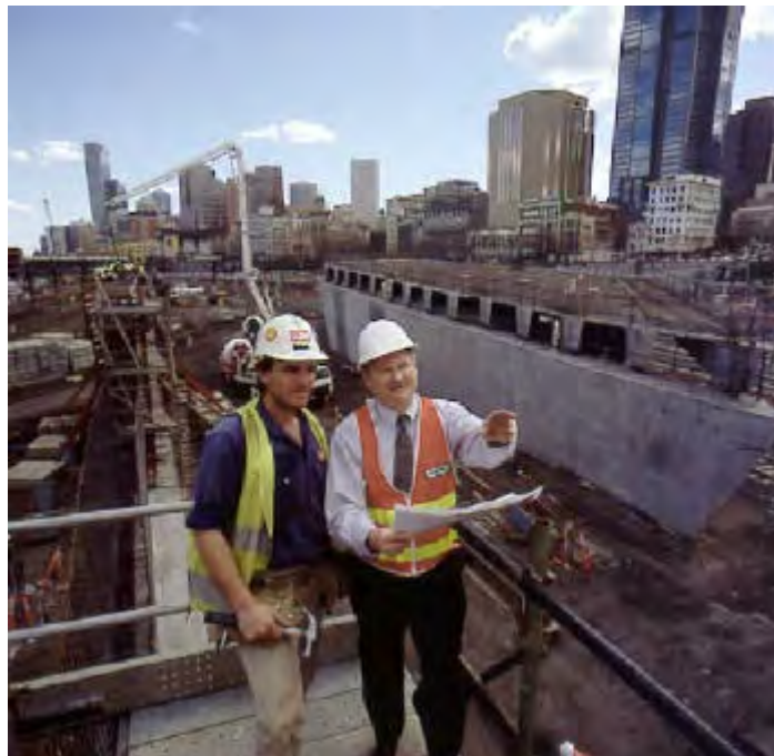
Road construction activities at the Exhibition Street Extension Project.
