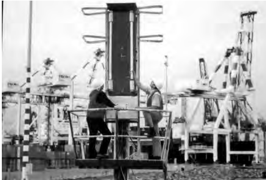
Inspection of mains-powered navigational aid.
