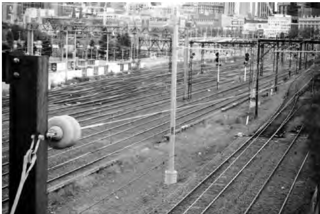
Rail infrastructure owned by VicTrack.
