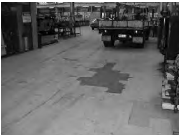
Floor of Building H.
