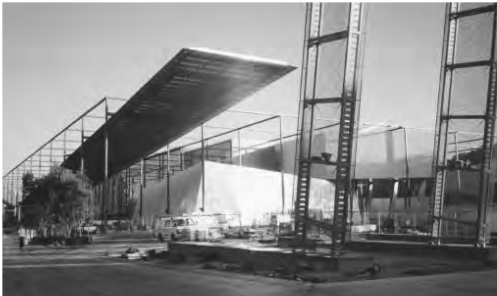
New Melbourne Museum complex, nearing completion.
