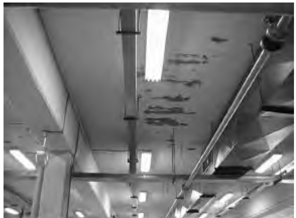
Ceiling of Building H.
