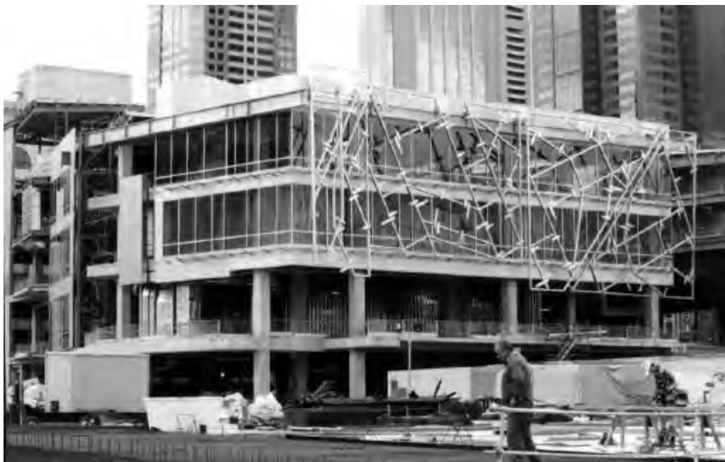
Façade of the Cinemedia Centre under construction at Federation Square.
