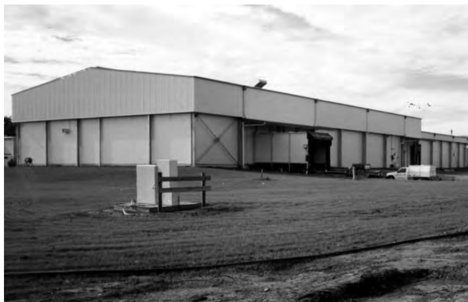
Export meat processing facility in the Colac-Otway Shire.
