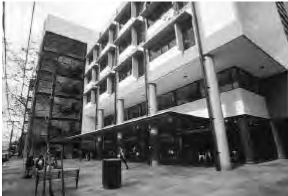
New Arts building in St John Street, Prahran.
