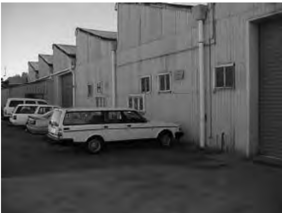
Rear of Building H.
