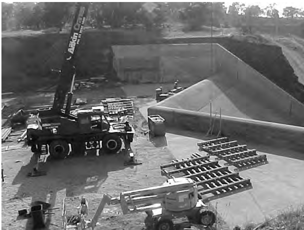
Construction works to improve spillway capacity at Rosslynne Reservoir, near Gisborne.
