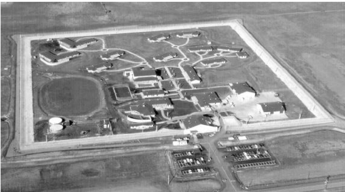
Metropolitan Women's Correctional Centre at Deer Park.
