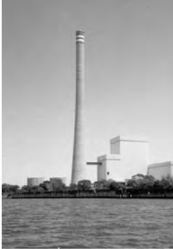
Industrial chimney stacks are used to reduce pollution at ground level.
