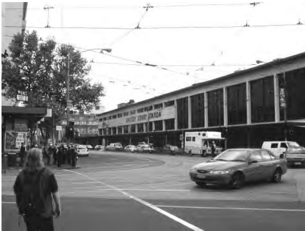
Existing Spencer Street Station site.
