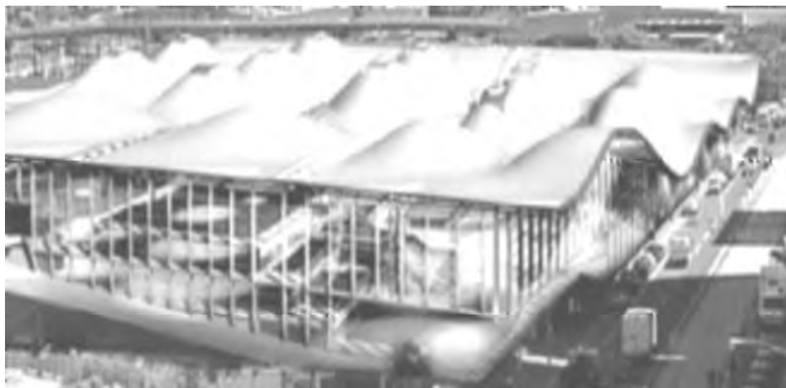
Proposed redevelopment of Spencer Street Station. (Photograph courtesy of the Department of Infrastructure.)
