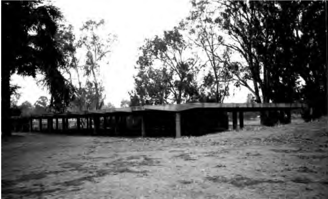
The partially constructed Lakeside Community Centre, located in central Benalla.
