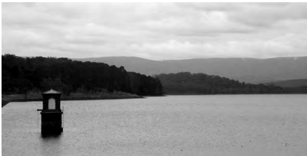
Yan Yean Reservoir has a total available capacity of 30 000 megalitres and supplies water to Melbourne's northern suburbs and central city area.
