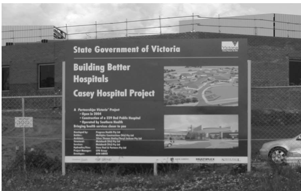
Commencement of the construction of the Berwick Community Hospital (now known as Casey Hospital).
