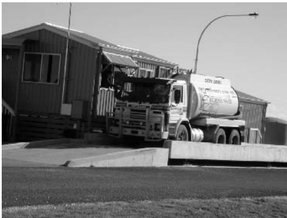
Newly constructed entry, office complex and laboratory on site.
