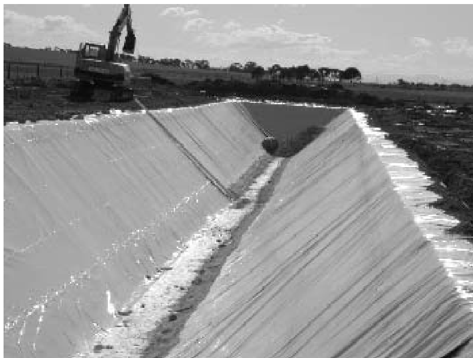
Landfill trench under construction being lined with geomembrane.
