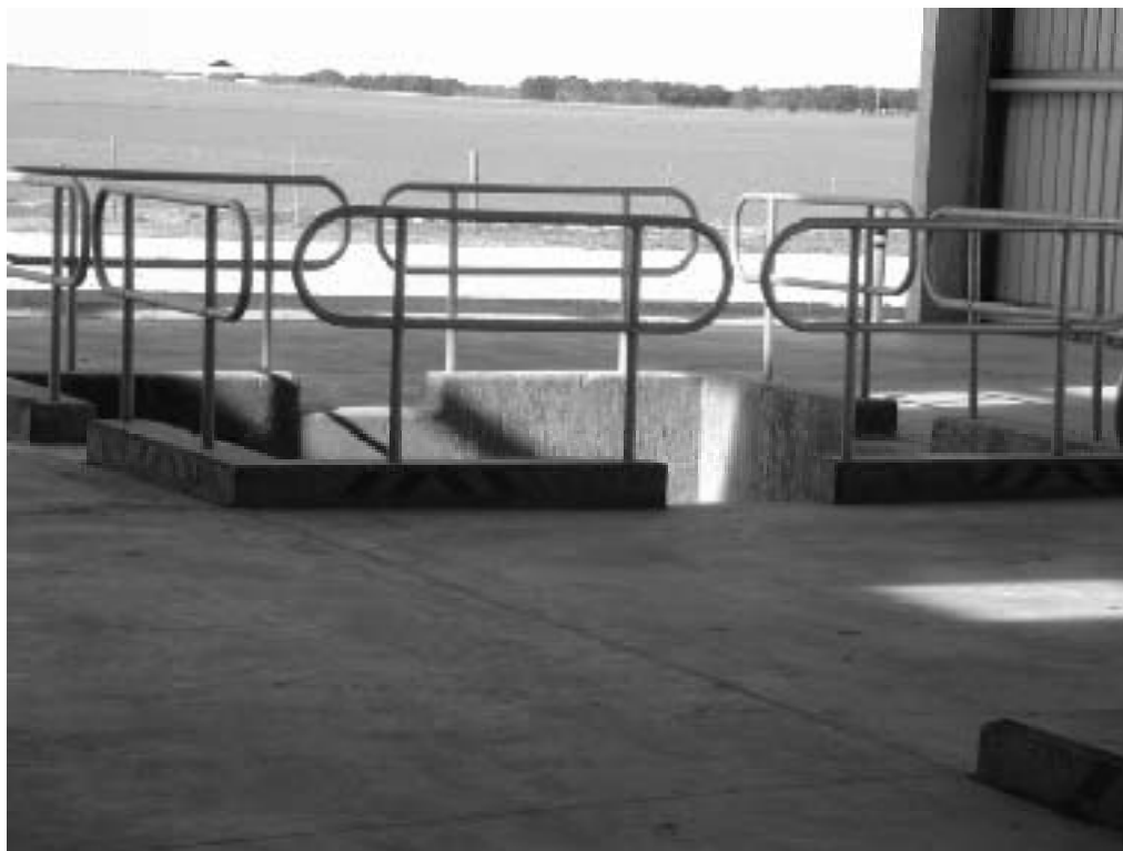
Recently constructed waste stabilisation pit.
