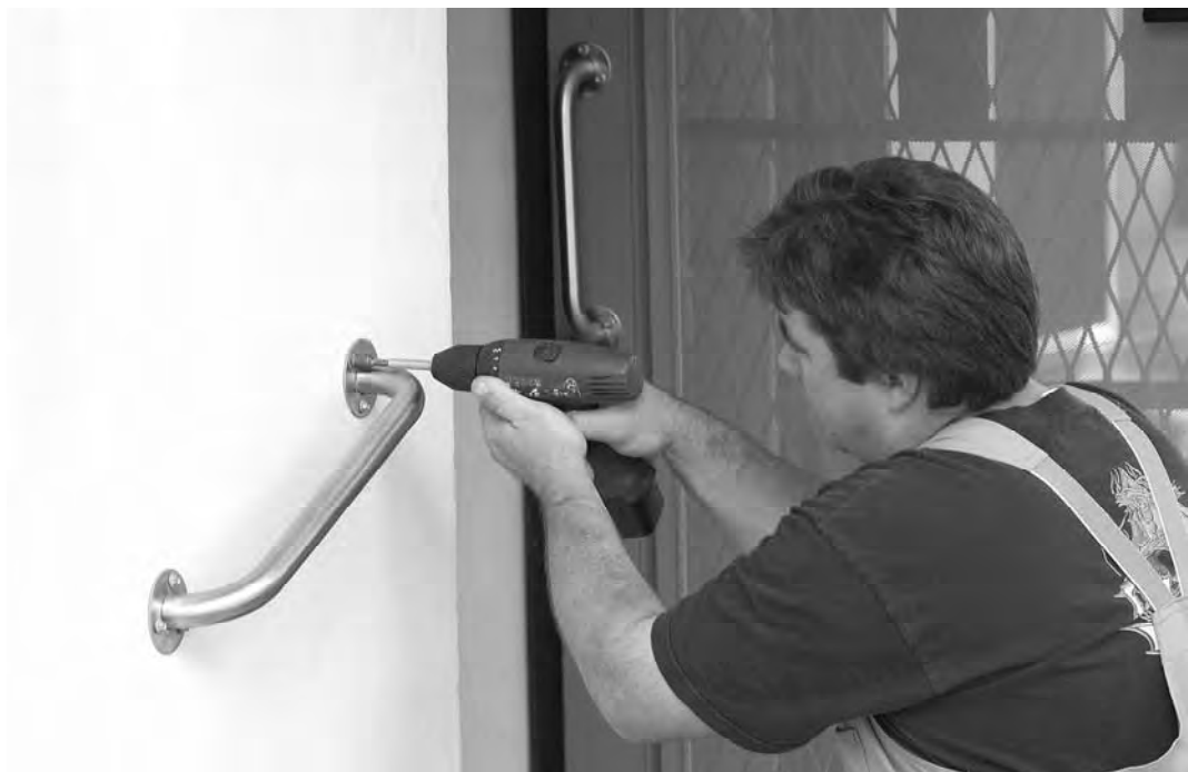
Workman installing a hand rail.
