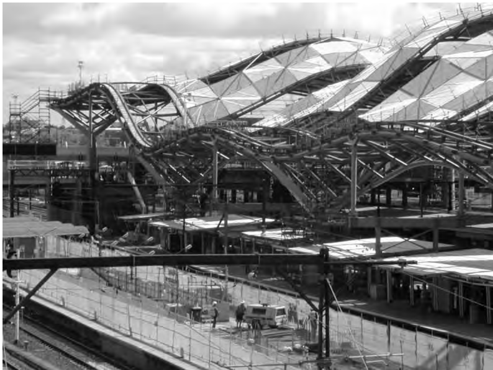
Spencer Street Station redevelopment works.
