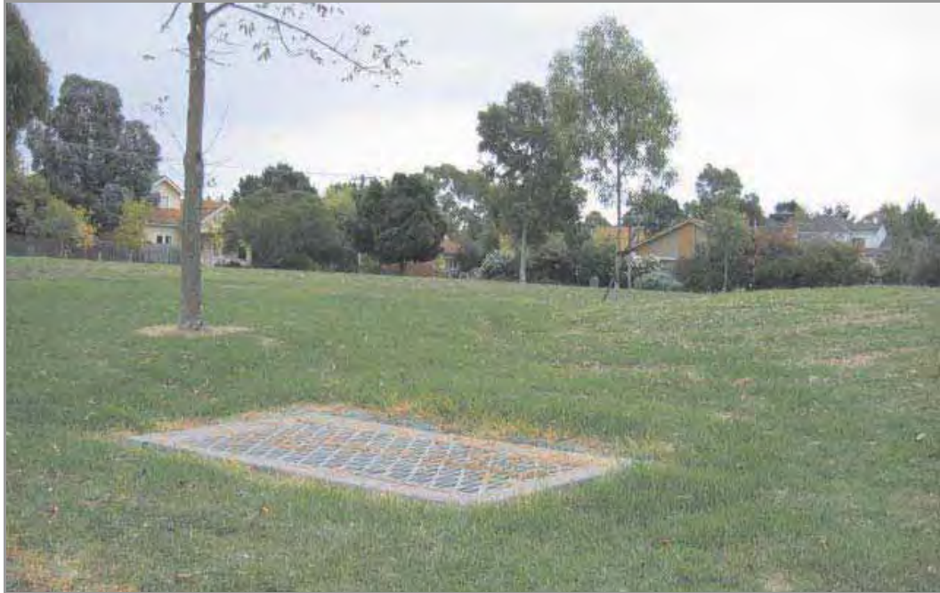
Stonnington duplicated its stormwater drainage pipe and connected into Melbourne Water’s main drain at this pit located in Daisy Park.
