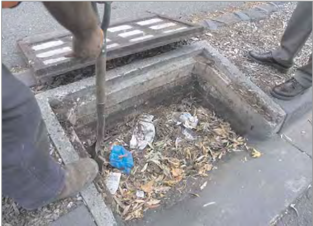
Boroondara staff undertaking routine maintenance of a stormwater drain.
