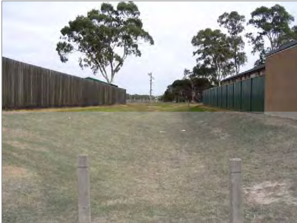
Overland flow path built into a new housing estate in Casey.
