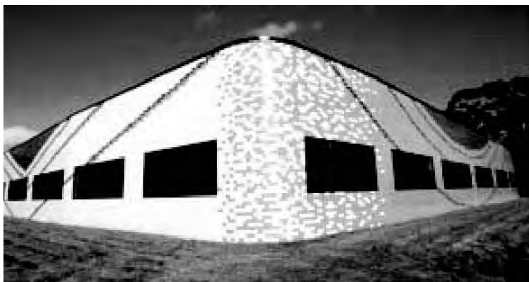
Centres for Information and Communication Technology were constructed in Bendigo and Ballarat using RIDF funds.
