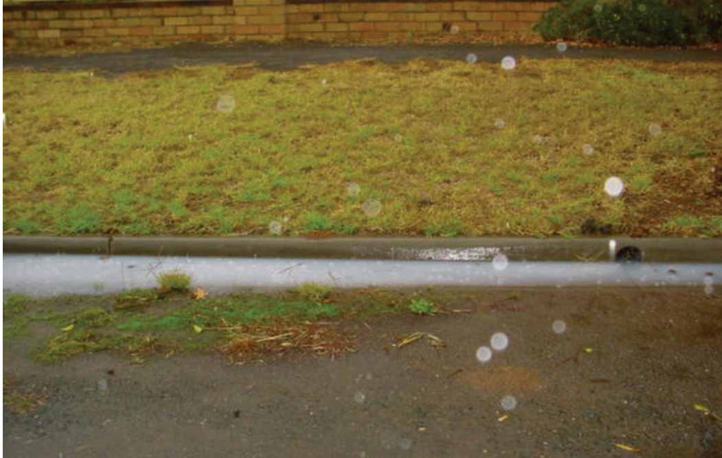
Greywater from poorly designed septic tanks flows into residential streets.
