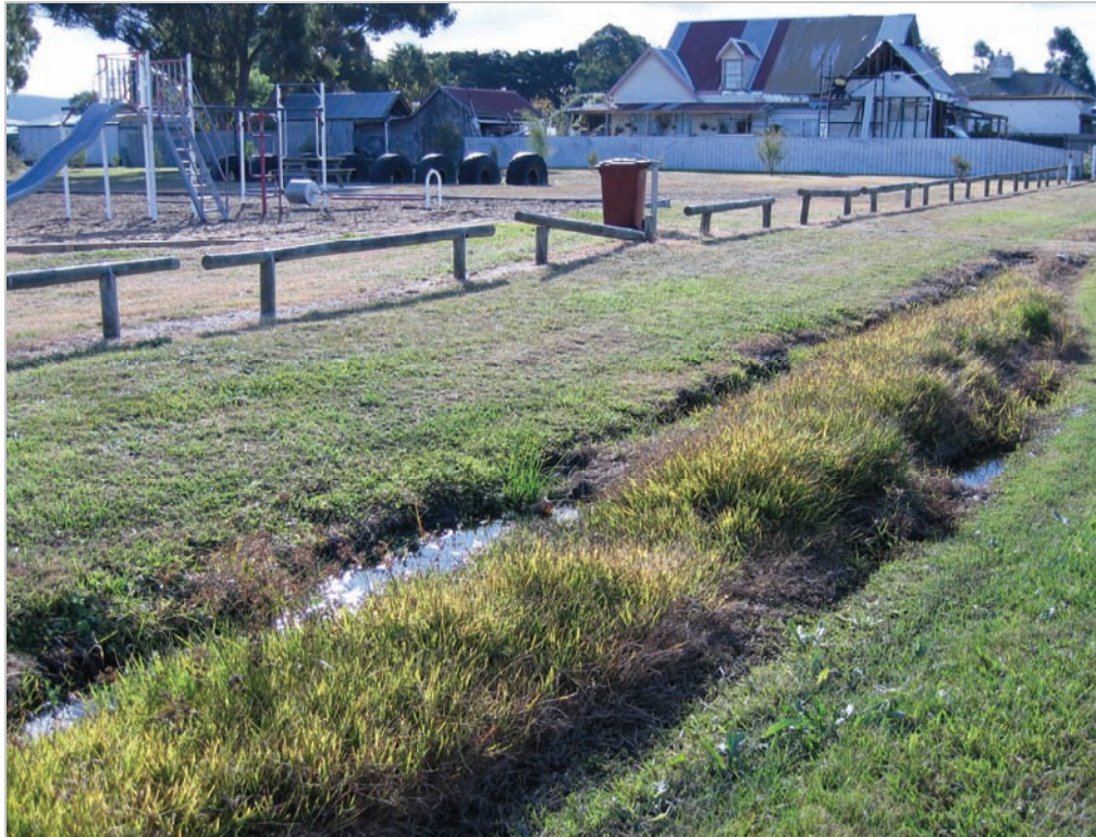
Open drains collect greywater adjacent to a children's play area.
