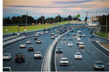
CityLink Tulla motorway. Photograph courtesy of VicRoads.
