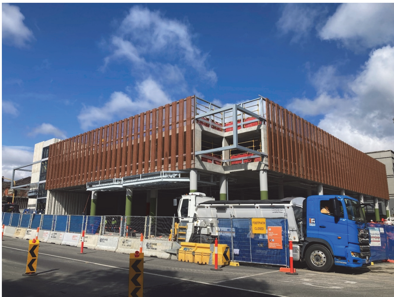
Figure 2: Greensborough Station multi-deck car park and bus interchange
