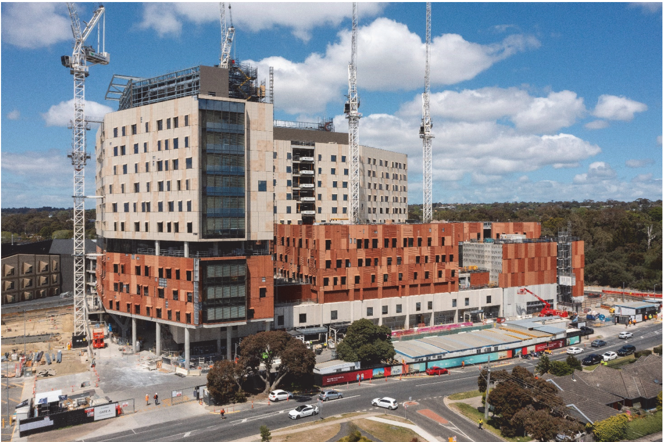
Figure 1: View of the Frankston Hospital redevelopment
