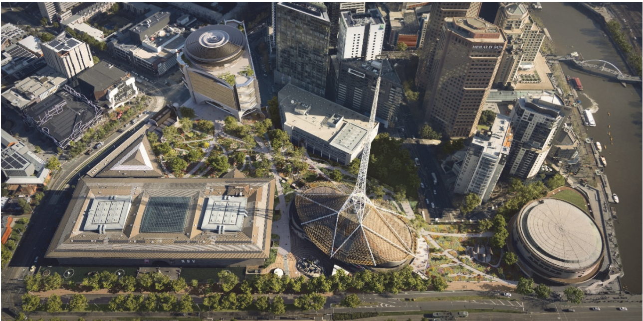
Figure 1: Artist's aerial impression of the Melbourne Arts Precinct Transformation Project Phase One when complete
