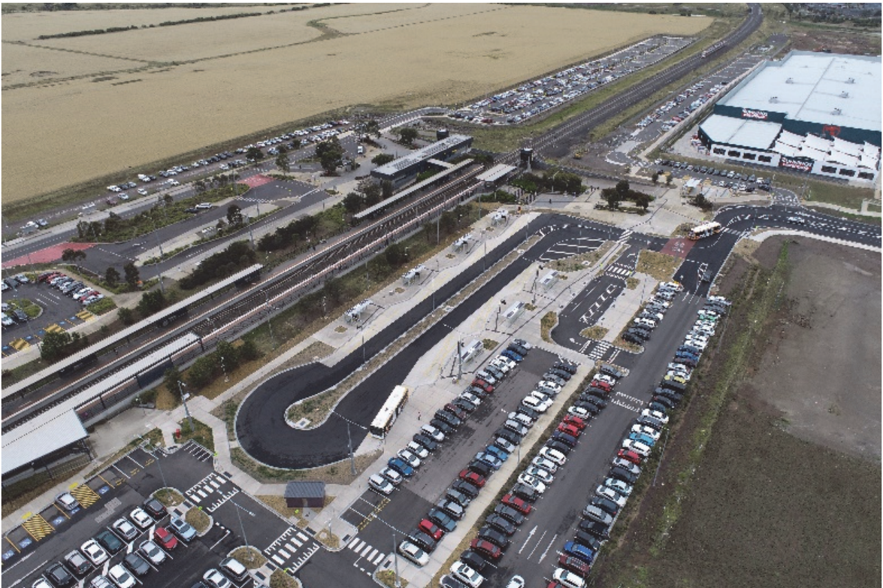
Figure 1: Tarneit Station car park and bus interchange
