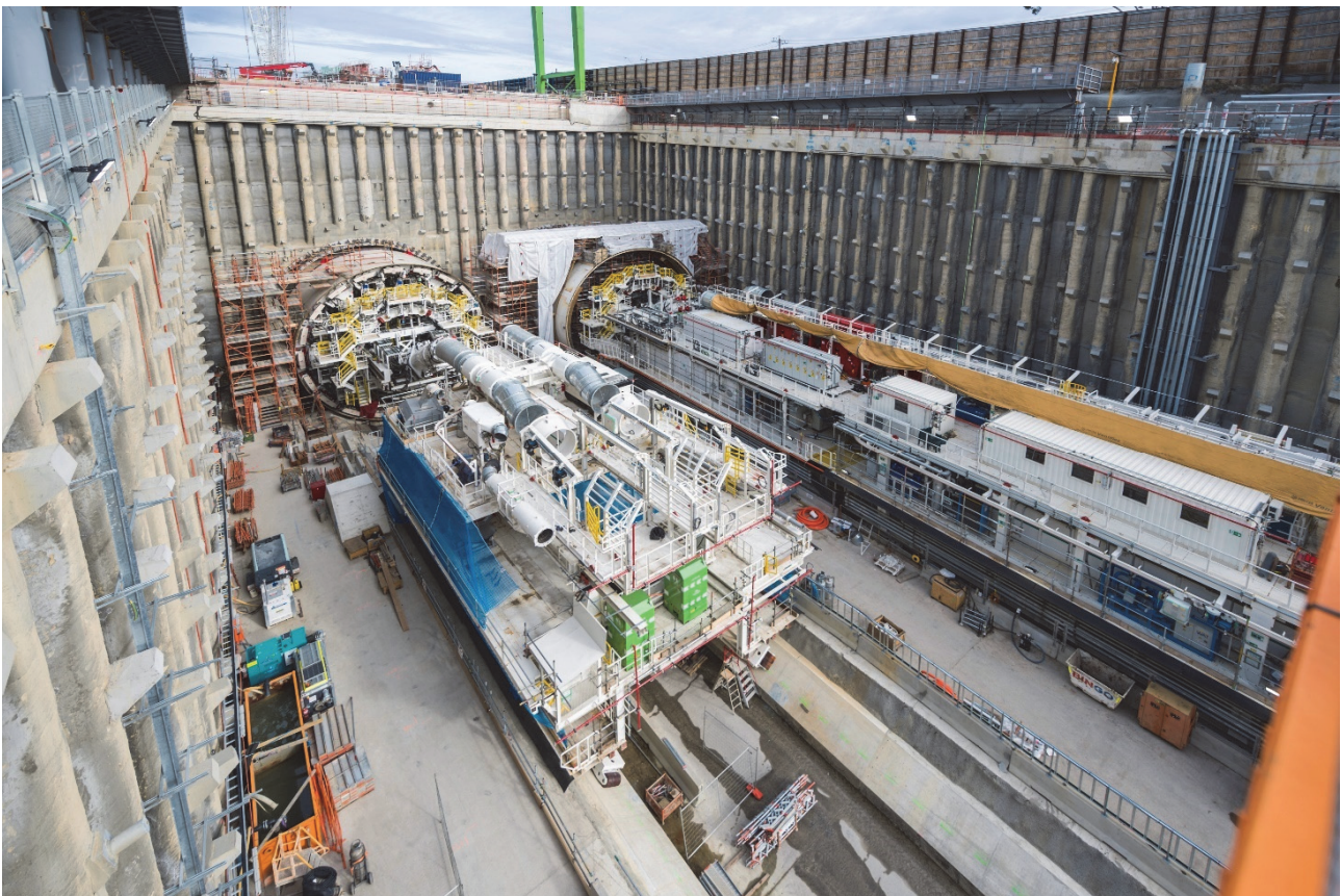
Figure 1: North East Link new twin tunnels construction
