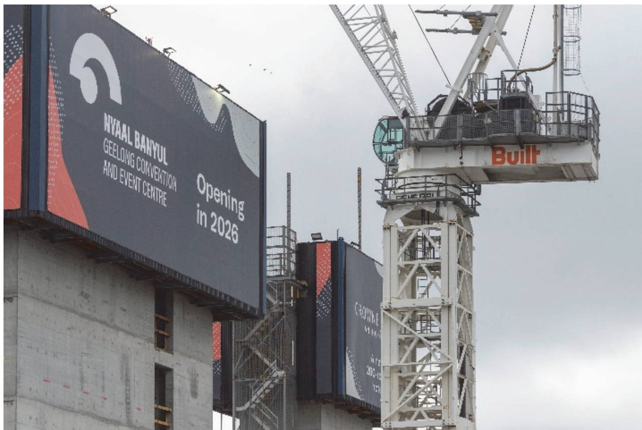
Figure 2: Nyaal Banyul lift cores under construction and site crane
