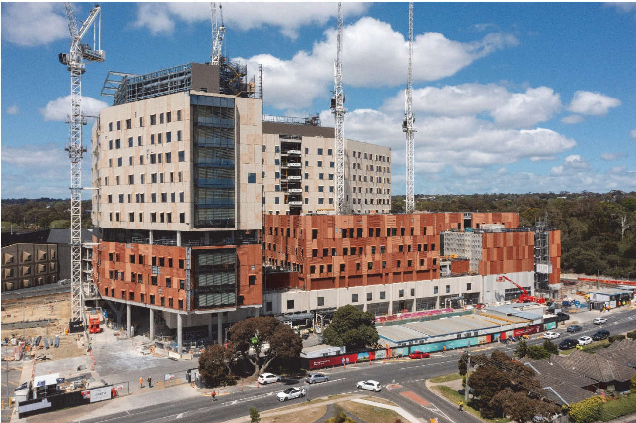
Figure 1: View of the Frankston Hospital redevelopment
