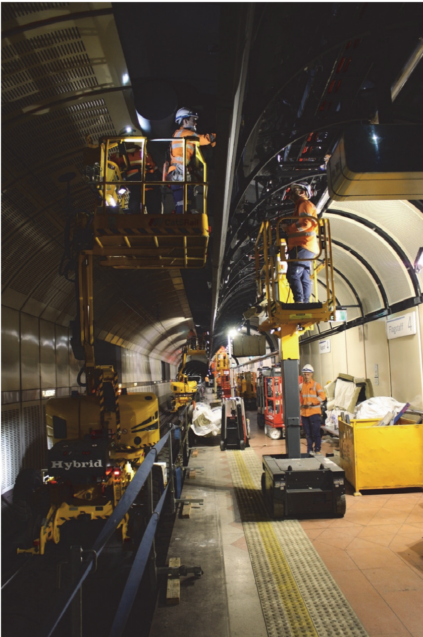
Figure 1: City Loop fire and safety upgrade in Flagstaff Station
