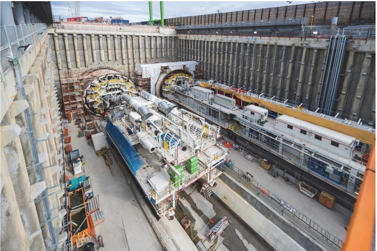
Figure 1: North East Link new twin tunnels construction
